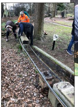
The club carries a small stock of serviceable sleepers for just this eventuality. As you can see from the pictures once the sleeper was removed all that remained were the anti-tip rails and signalling conduit
