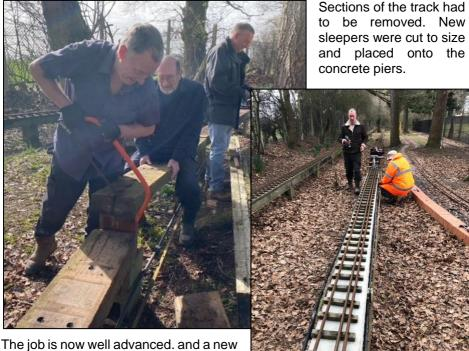
The job is now well advanced. and a new concrete screed laid (see front page) before the track could be installed.
